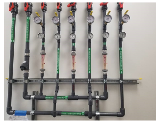
Figure 10: Cooling water pressure check
