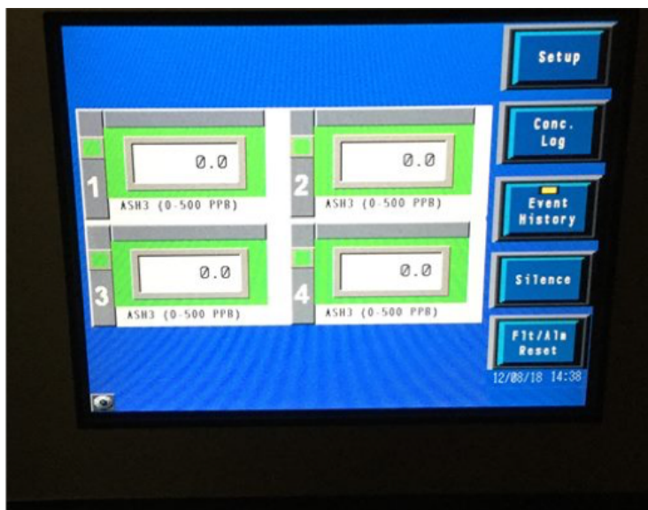
Figure 3: Gas sensors outside the lab door
